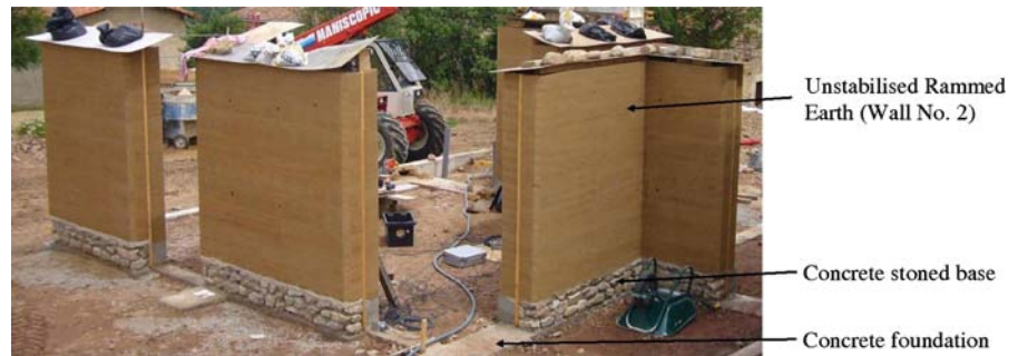
Fig. 2 Rammed earth house under construction, at the time of the first measurements, in June 2006
